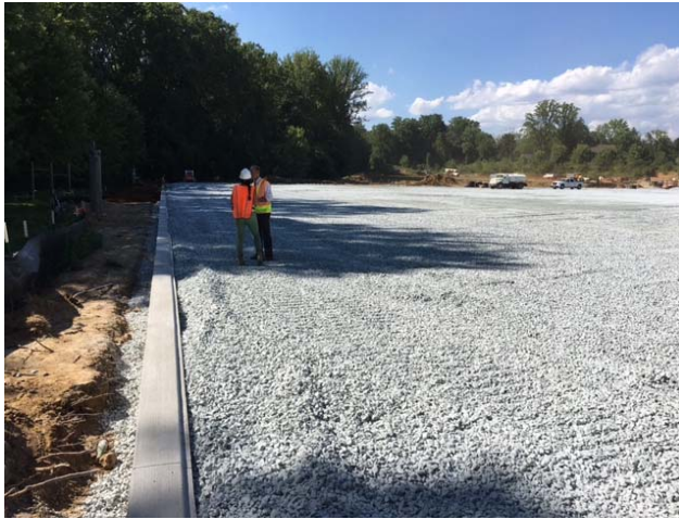
Stone Sub-base and Perimeter Concrete Nailer Installation for Synthetic Turf
